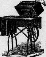
Rotary Hook, Straight Needle, Independent Take Up, Loose Pulley and Improved
