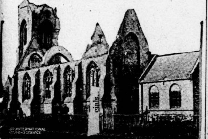
Exterior of the church at Ramscapele after the once beautiful edifice had been wrecked by the shells of the contending armies.
