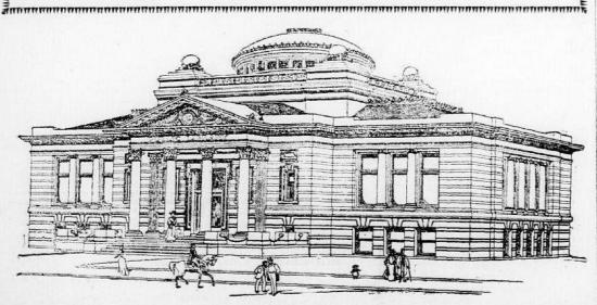
The Carnegie public library in the city of Fort Dodge, Ia., is in course of erection, and will be completed about July 1 of this year. The plan of the building is in the form of a cross with a dome in the center. The width of front is 91 feet by 72 feet deep. The main entrance vestibule is on a level with the portico floor. There are mer-ble stairs to main and basement floors. On the main floor are located the de-livery room, with glass dome ceiling
