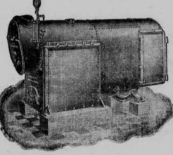
The "ECONOMIC" return Tubular Portable Boiler. It is self contained, and readily removable from place to place. excellences of a well et stationary boiler
