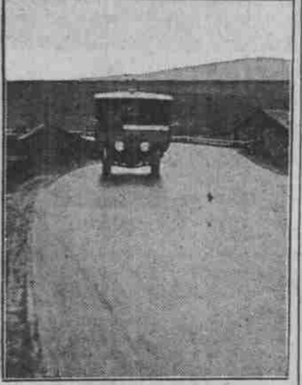
Hard Surface Road Built by Federal and State Funds.
