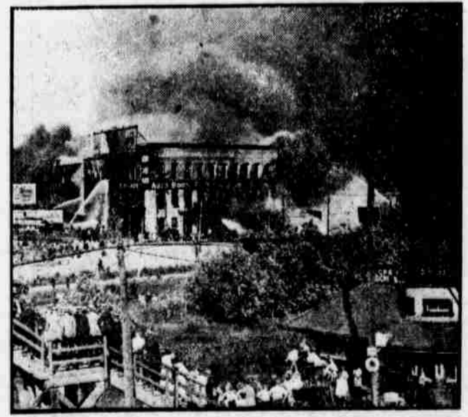
(By Pacific & Atlantic) Conboy building, first concrete structure built in Toronto, Canada, was destroyed by fire, despite long battle with flames. It was built in 1902.
