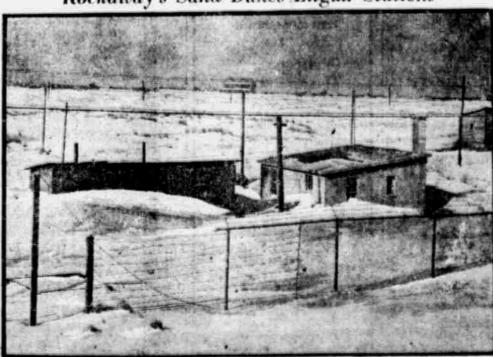
Shifting sands all but buried government pumping station at Rockaway Point, N. Y., during the winter. To repair machinery, roof and part of side of one of the houses had to be removed. (Copyright: 1924: Pacific & Atlantic Photos, Inc.)
