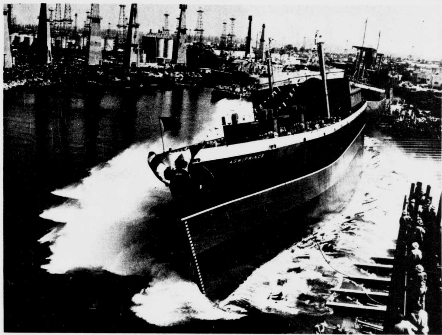
Lifeline of the anti-axis defense—ships and more ships. Here the 12,000-ton cargo ship Agwiprince hits the harbor water at Long Beach, Calif., with a great splash in a broadside launching. Her 14-knot speed would give her a big advantage over U-boats.
