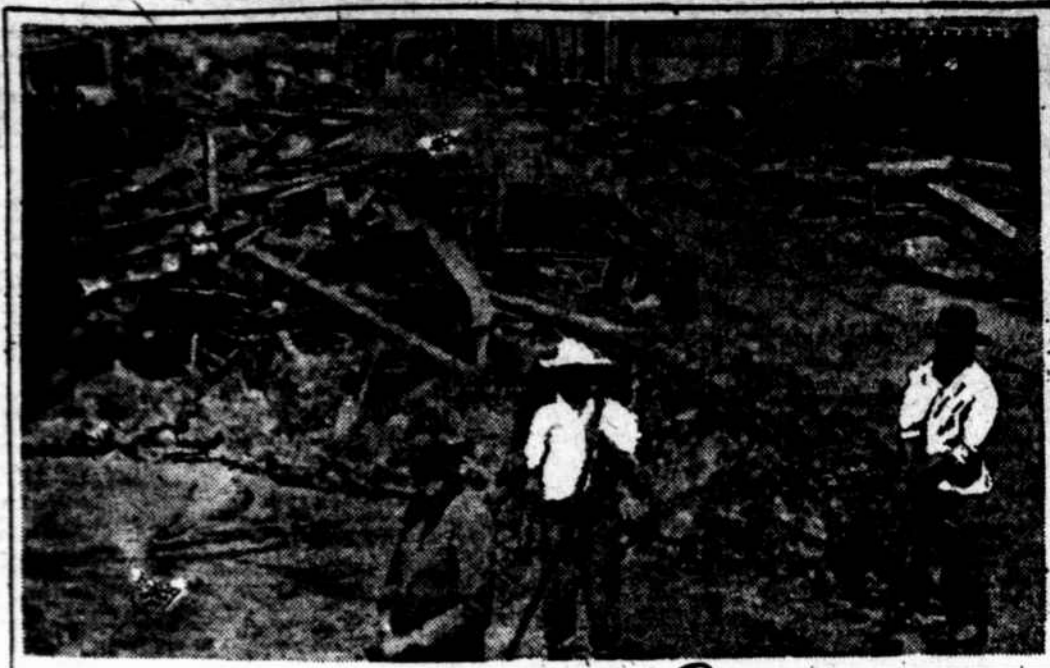
Chapparral street in Corpus Christi, Tex., the day after the big storm, was filled from end to end with a mass of debris. Mexicans here are at work cleaning up the wreckage.
