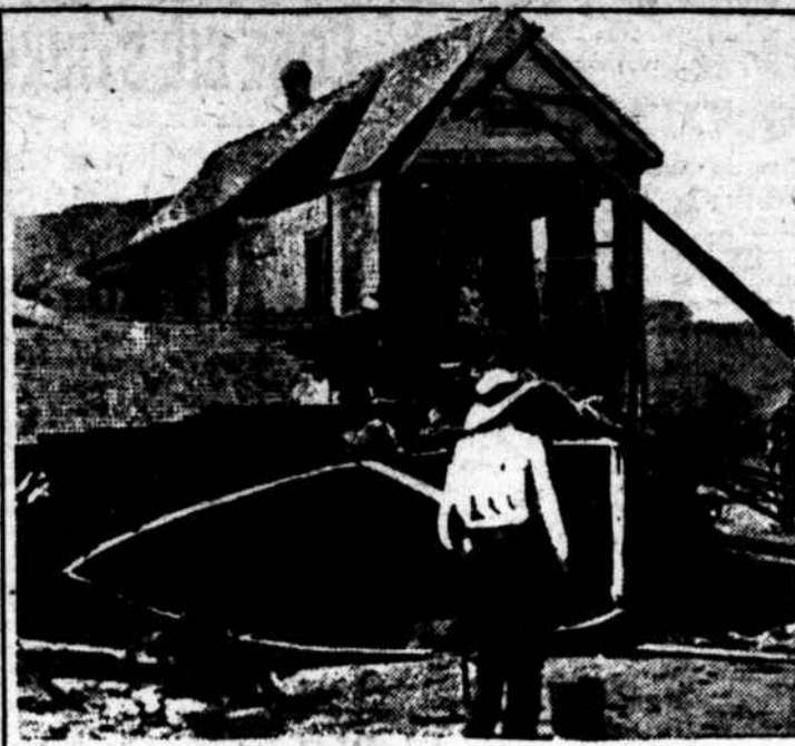
This house was lifted by the hurricane and flood that struck Corpus Christi and deposited on top of the boat part of which is seen in the foreground.
