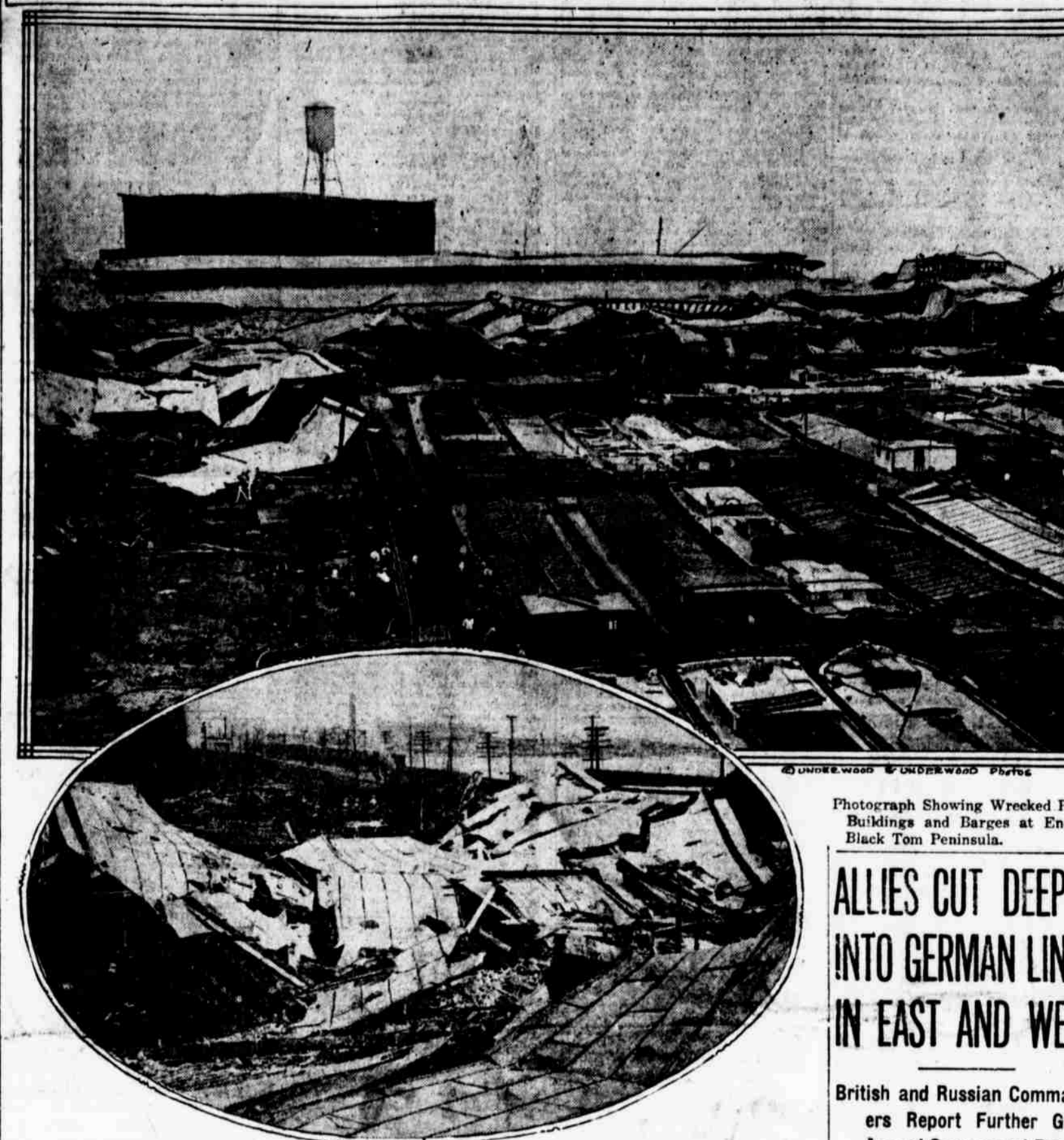
Ruins of Thirteen Warehouses of the National Storage Company, Leveled by Yesterday's Explosion.
