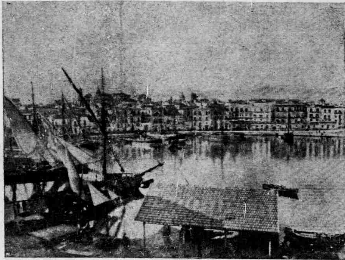
"LA CALA," PALERMO (THE OLD HARBOR), PARTIALLY RUINED BY THE GREAT EARTHQUAKE.
