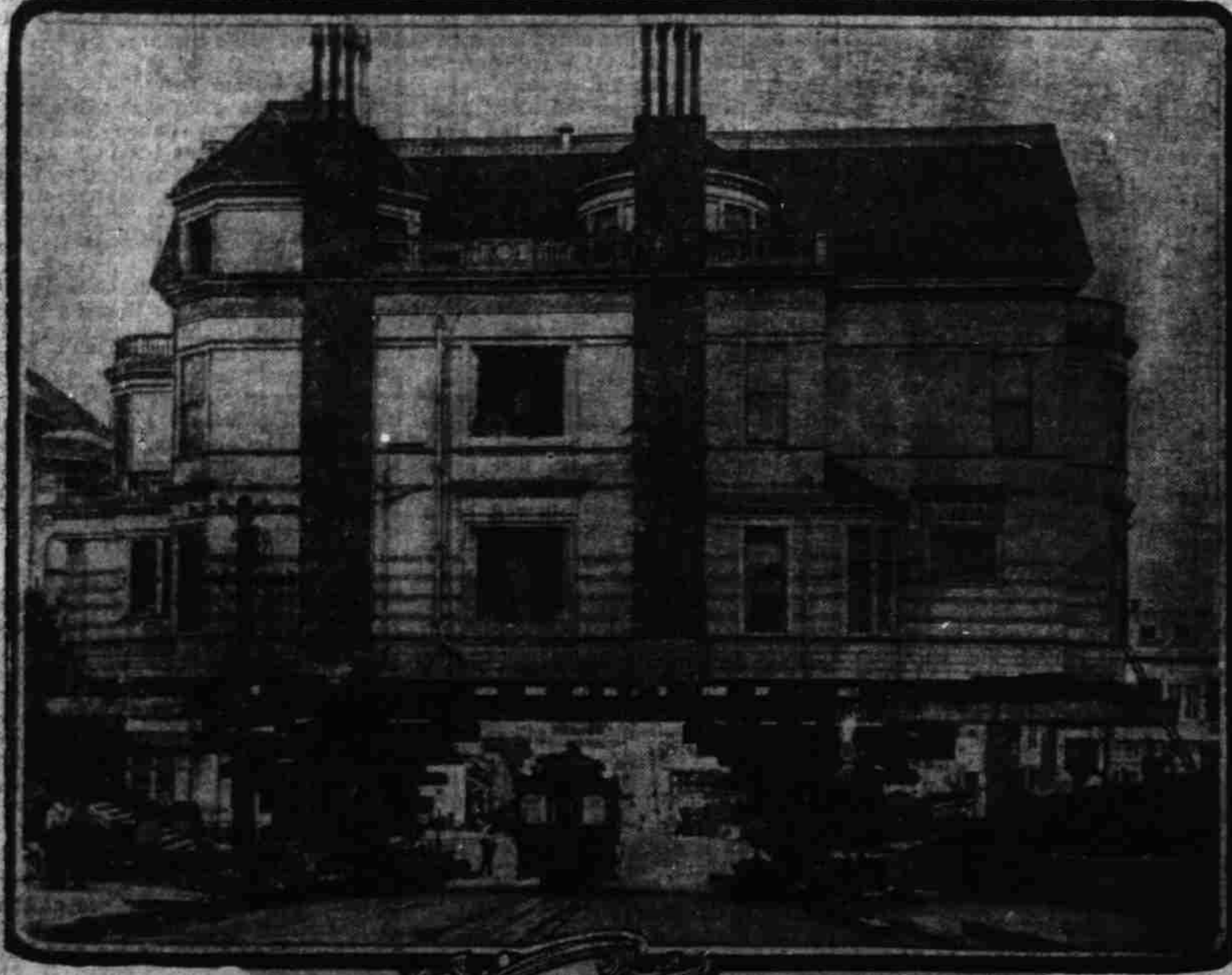
Among the many freak engineering stunts for which San Francisco is famous the above picture, photographed especially for the Honolulu Star-Bulletin, is regarded as one of the most striking. A large old-fashioned house is being moved to make room for a modern structure and it is necessary to block the entire street in order to move the house. However, Jackson street is a cut-line street and it was not desired that transportation be closed, consequently the house was placed on skids to such a height that it is possible for the cars to proceed underneath, as is clearly shown in the picture.
