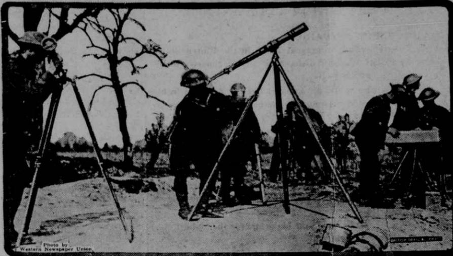
It is an exceedingly technical task to determine the attitude and speed of a fast-moving enemy plane. Here members of a British anti-aircraft section are getting the range of a German Gotha; in turn they will communicate it to quick-fire guns along the line.
