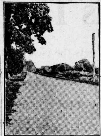
Ohio State Highway, Brick.
