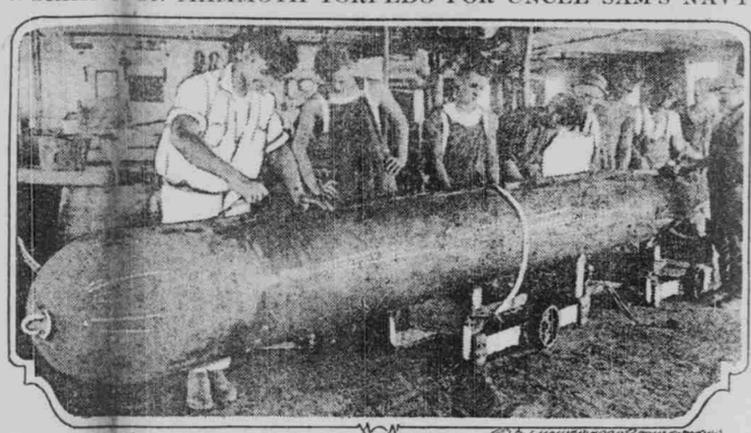
One of the giant torpedoes destined for use on American battleships in process of assembly. Torpedoes for the navy are shipped in parts from the factory at which they are made to a barge moored in a little port somewhere along the coast. Here they are assembled and then tested. Government officials watch the tests carefully and reject all torpedoes found not up to the standard. This photograph was taken inside the barge while the torpedo was being put together.
