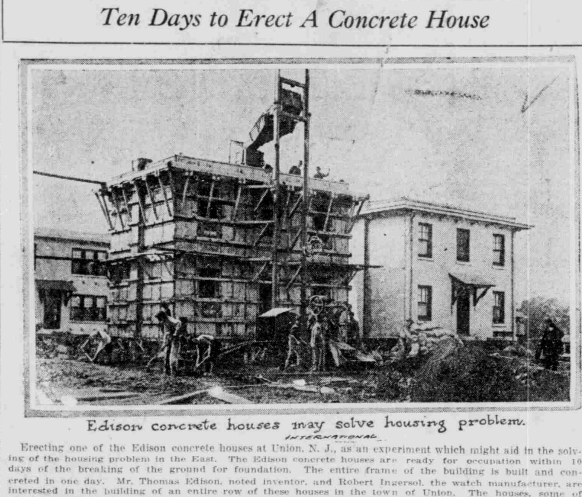
Edison concrete houses may solve housing problem.
