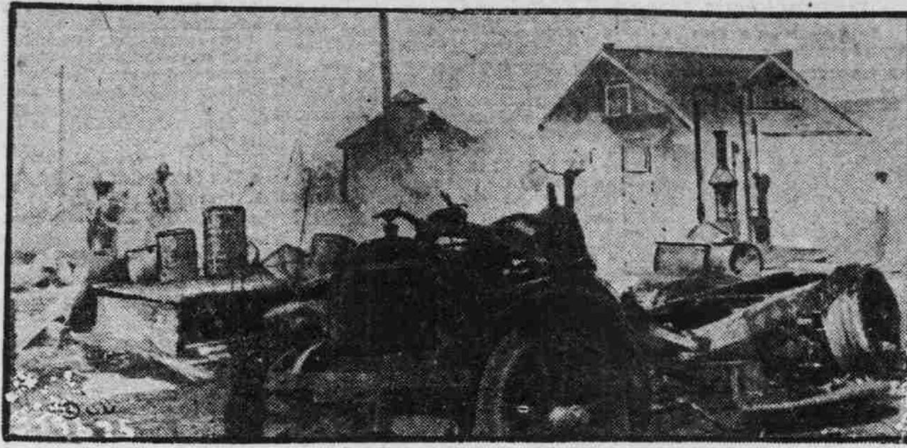
All that is left of gasoline truck and station after explosion. Eight persons were killed, a gas station and gas delivery truck were destroyed when a worker with a blow-torch came too close to the gas tanks at a station at Downey, near Los Angeles. Tanks and oil drums were hurled hundreds of feet by the explosion.
