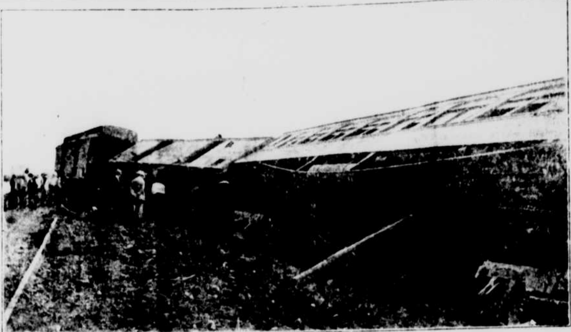
TRAIN 123 IN THE DITCH AT OSPUR.
