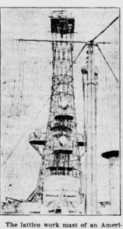
can battleship from the top of which the fire of the guns is controlled.
