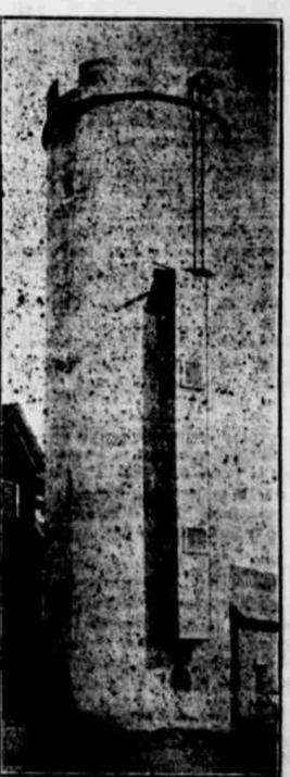
POLK SYSTEM SILO. 16x60-Foot Silo With 25,000 Gallon Water Tank on Top. Total Height 86 Feet.
