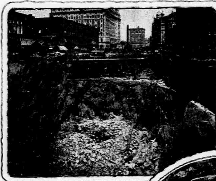
In This Hole the Subway Intersects the Cellar of a Skyscraper Since Erected
