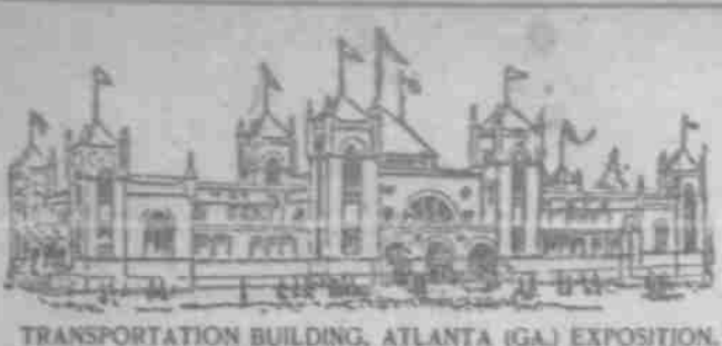
TRANSPORTATION BUILDING, ATLANTA (GA.) EXPOSITION.
