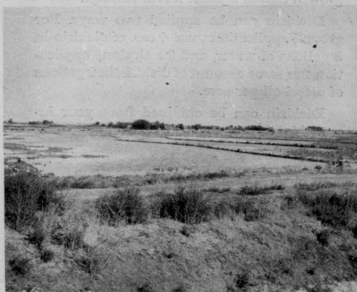
This picture shows some flooded basins in action leaching out excessive salts and alkali. The basins are made by constructing contour dikes across the fields. It requires a year and about five leachings to reclaim the land.
