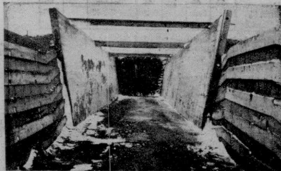
This side-hill silo on the John Horst place, Dawson County, was filled with corn silage. The silo is an ideal type of concrete construction.
