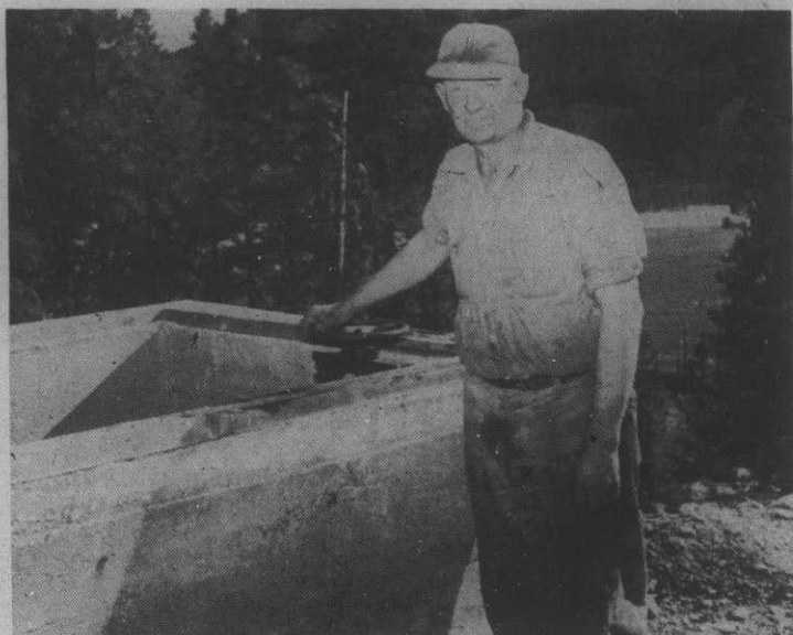
Otto C. Hansen, Mineral county stands at the gate wheel in the key drop box in his irrigation system. Water released here plunges down steel pipe line for a 180-foot drop to his fields below developing 70 pounds pressure for operation of sprinkler system. The mountainside creek formerly sank into an underground channel passing under the farm lands and into the river eventually.
