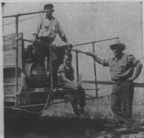
Jergen Dokken, Valley county, sprayed about 400 acres of his spring wheat this year using the tractor-drawn trailer with 42-foot boom seen above. Two swivel wheels were added for stability to the trailer in place of one that came with the original machine. Power take-off of the tractor operates pump developing 35 pounds pressure for the nozzles spaced every 20 inches on the 42-foot boom. He was applying 3/4-pint (3/10 pound) of 2,4-D ester per acre in 5 gallons of water at a speed of 5 miles per hour. The tank holds 300 gallons and is filled about 3 times a day for spraying on from 120 to 200 acres per day.
