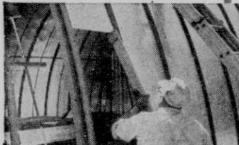
Steel sheets slide into place—are bolted into a one-piece steel shell.
