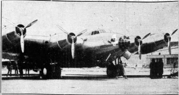
MIGHTIEST, more formidable than any other fighting aircraft, here is Uncle Sam's newest 20-ton bomber as it was wheeled out on Boeing field, Seattle, Wash., for a test. It has been under construction for three years, so carefully guarded that only a few air corps officers know its specific details. It is 75 feet long and has a wing spread of 105 feet. It carries a ton of bombs at 252 miles an hour.
