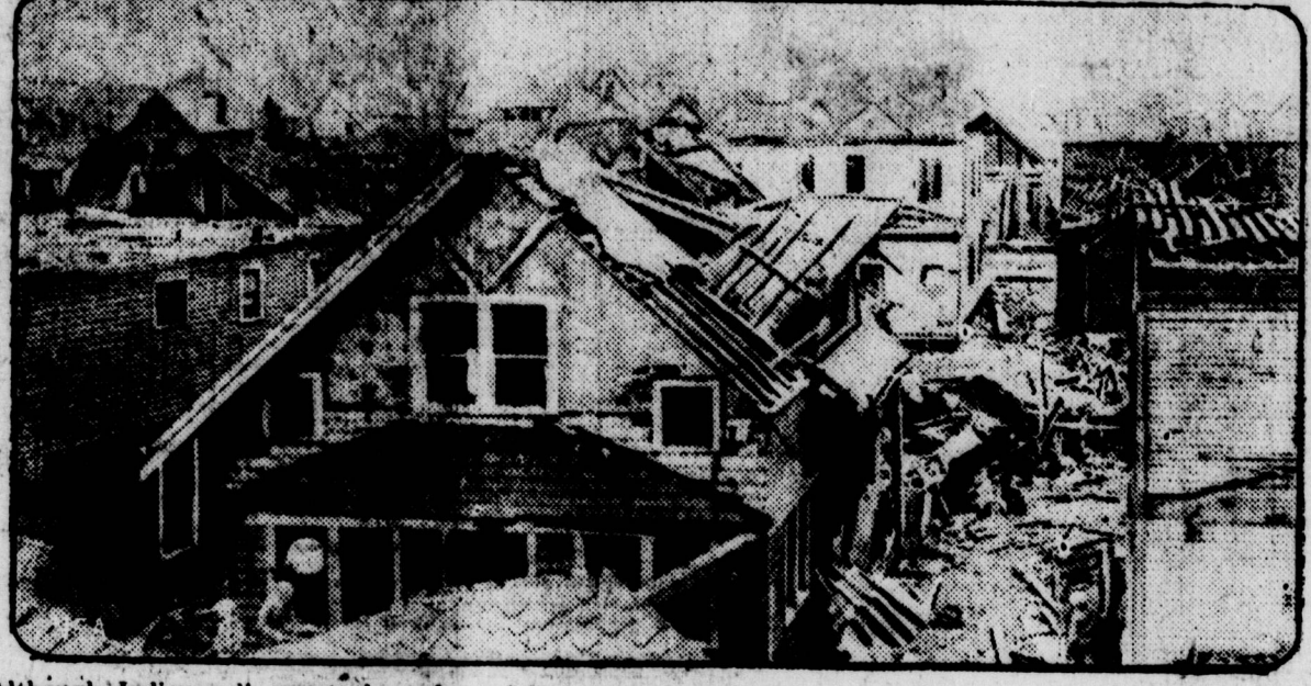
Although Indianapolis went through a violent tornado without loss of life, houses in certain residence districts looked as if they had been under shell fire. This shows a section of frame dwellings unroofed and battered by the howling wind, which struck just at dusk and without warning.
