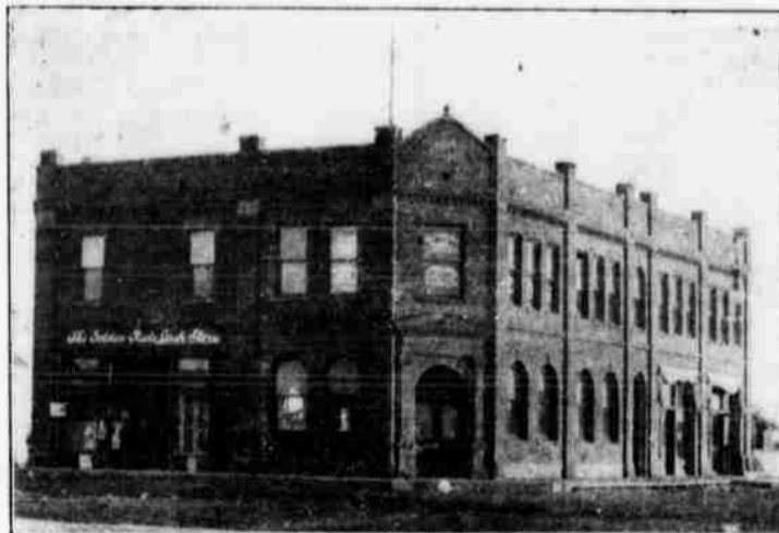
FIRST NATIONAL BANK BUILDING, TUCUMCARI, NEW MEXICO.
