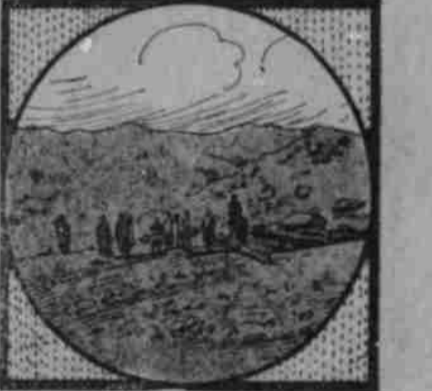
Native Miners Sinking a Shaft.
