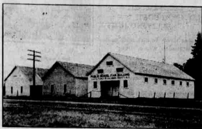
FAIR GROUND BUILDINGS
