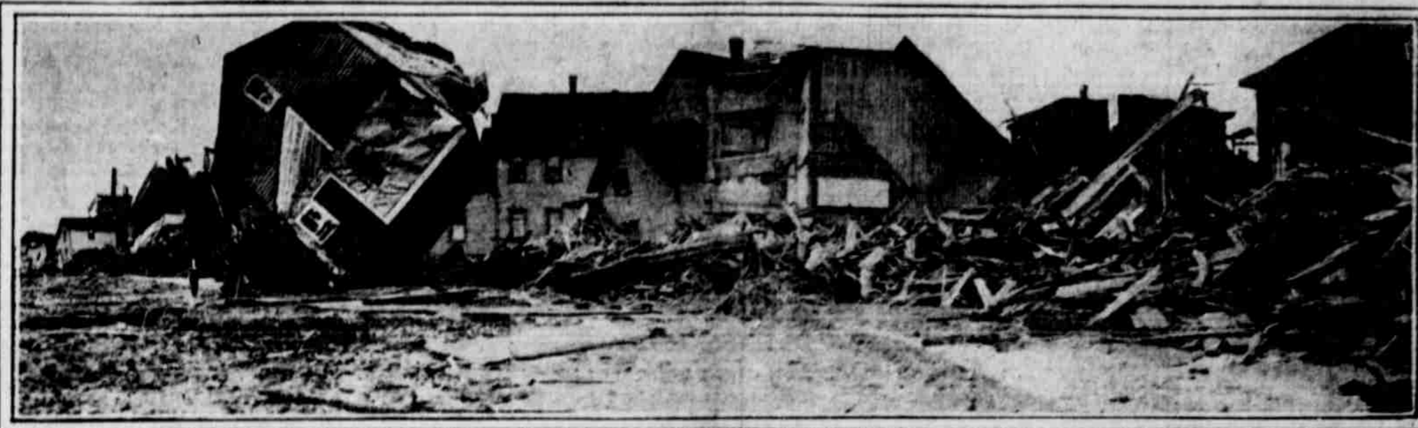
RUINS IN OUTSKIRTS OF OMAHA. In this picture is shown an actual scene in Omaha, Neb., following the great cyclone which caused so much damage and loss of life. The destruction shown here is only a small part of the devastation caused by the awful storm.
