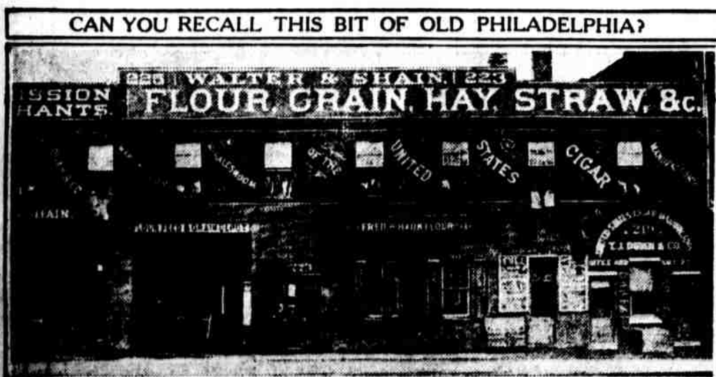
A BIT OF NORTH BROAD STREET IN 1880. Imagine any one trying to buy flour, grain and hay along automobile row today. These buildings were located between Race and Vine streets. Miss Irene E. Dunn is the contributor. If you have an old Philadelphia photograph, please send it to the EVENING PUBLIC LEDGER
