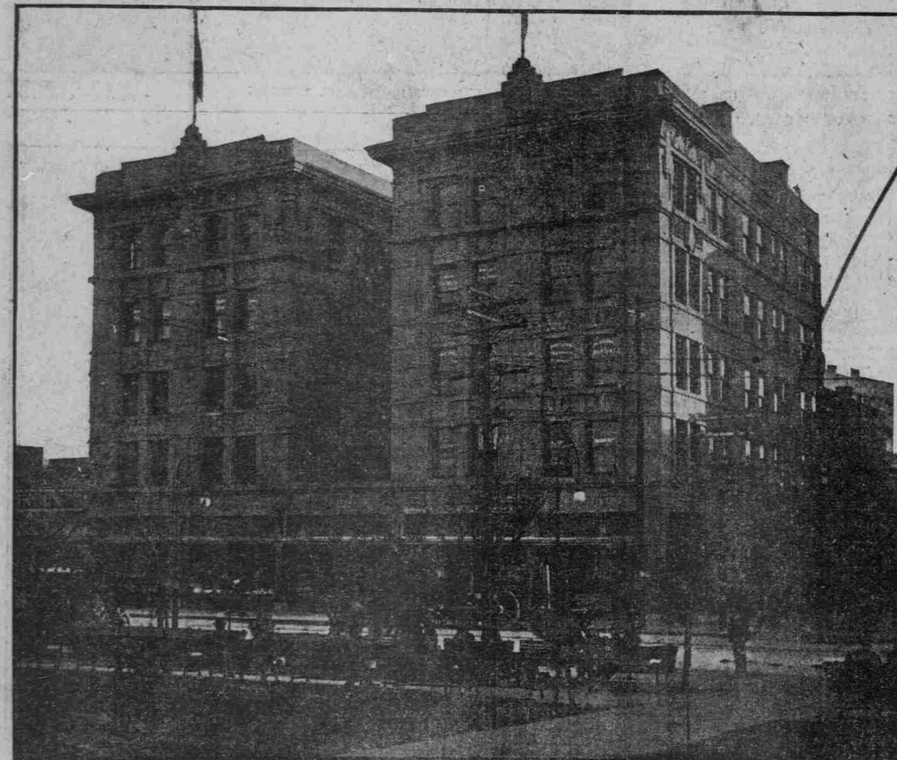
Sorenson & Morgan, Contractors.
