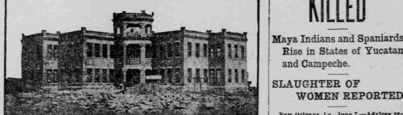
Alpine, Texas, high school, now nearing completion. One of the costliest school buildings in Texas. The Alpine Normal school will be held there this summer.
