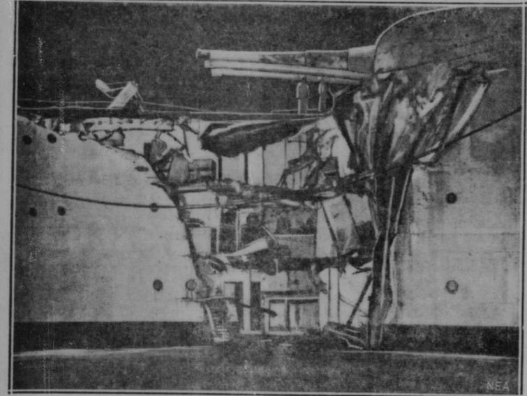
With three officers dead and a gaping hole, 40 feet wide, torn in her prow, the U. S. cruiser Chicago limped into Mare Island navy yard in San Francisco Bay after a collision with a British freighter. Damage is shown above, where the prow of the freighter plowed through armor plate to almost amidships and scraped one of the guns, pictured near top. A "ghost ship" is sought, officers declaring that it loomed out of thick fog to throw the cruiser off her course, into the collision.
