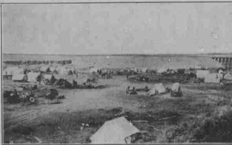
CONSTRUCTION CAMP, OASIS COMPANY, AT RIVERSIDE, UTAH.
