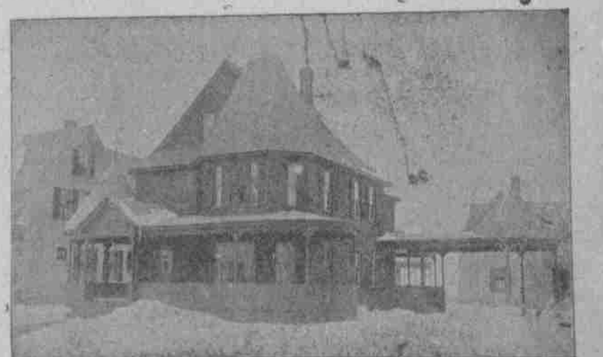
RESIDENCE OF J. W. GORDON, RICHARDSON STREET.
