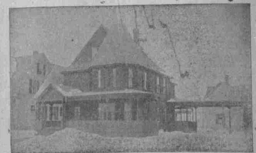
RESIDENCE OF J. W. GORDON, RICHARDSON STREET.
