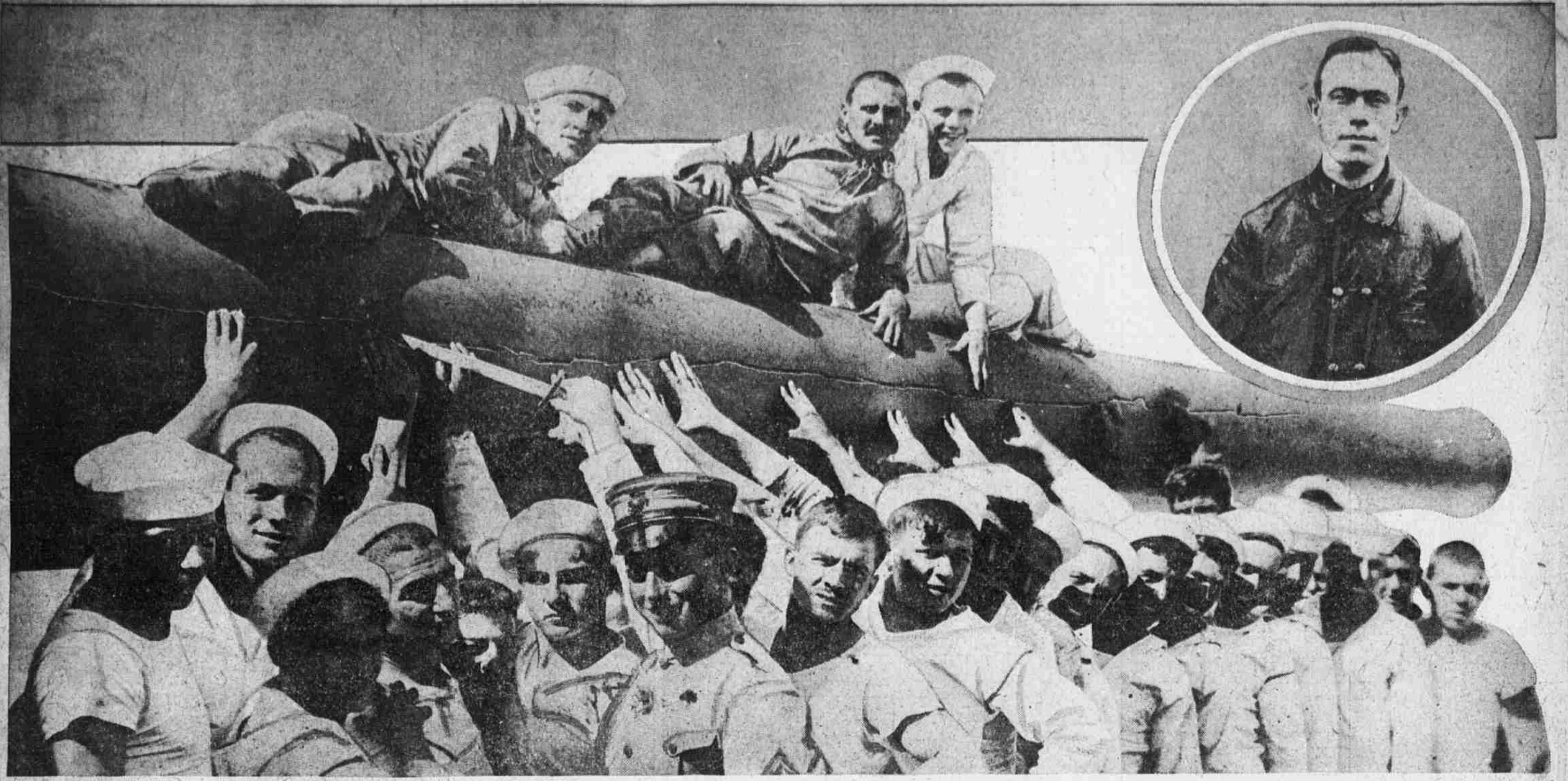
EXCLUSIVE PHOTOGRAPH SHOWING HOW 12-INCH GUN ON BATTLESHIP MICHIGAN CRACKED ALONG VIRTUALLY ITS ENTIRE LENGTH IN RECENT FIRING PRACTICE OFF GUANTANAMO BAY. As a result of the discovery of this defect, all four big guns in the forward turrets have been discarded and new ones are being mounted while the ship is undergoing repairs at the Navy Yard. Above, to the right, is Lieut. H. A. Dargue, who was knocked unconscious in the wreck of the sixth United States aeroplane in Mexico. He had to walk 65 miles back to camp. His home is in Ridgewood, N. J.
