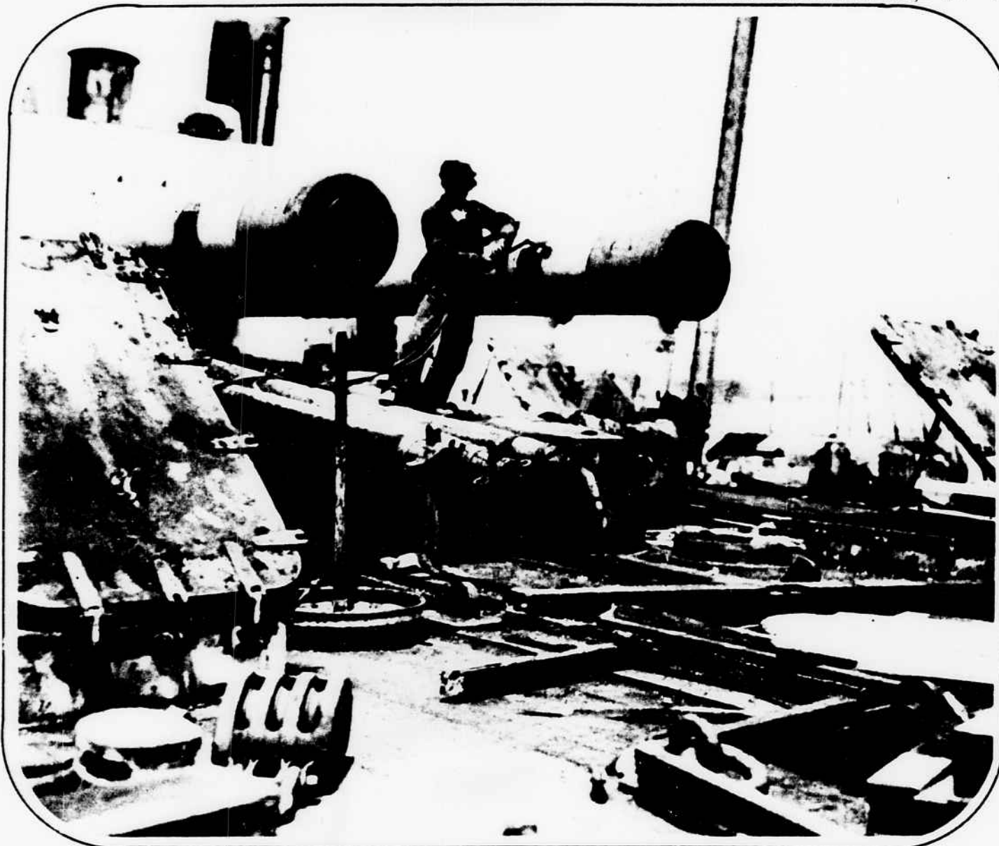
Scrapping some of the great ships of Uncle Sam's Navy at Philadelphia. Photograph shows work on the battleship Maine. The workman is cutting holes in the 12-inch guns. ©P. & A. Photos
