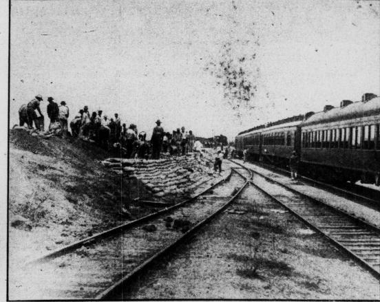
BATON ROUGE FIGHTS FLOOD THREAT AS CREST DESCENDS. Workmen throwing up sandbag reinforcements on the Mississippi River levee along the water front of the Louisiana city, in an effort to protect the railroad tracks from flood waters. High winds and stormy weather have added to the danger at this point along the Mississippi during the past 24 hours, as the levees face the attacking flood crest. Copyright by P. & A. Photos.
