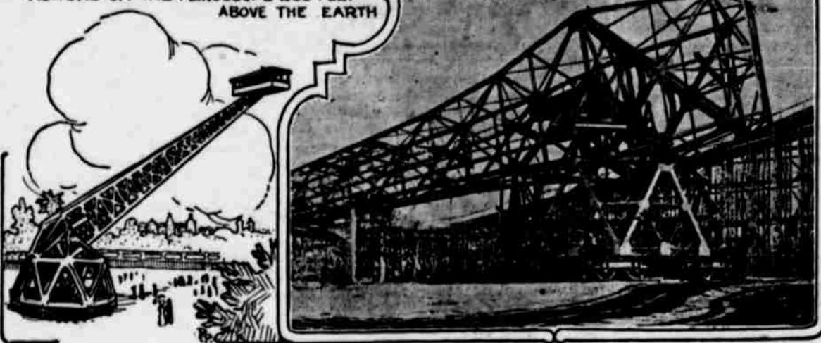
THE GIANT FRAME OF THE AEROSCOPE AS IT APPEARED UNDER CONSTRUCTION
