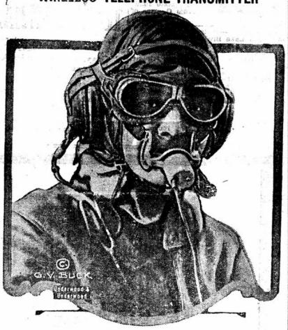
This is the transmitter of the wireless telephone that has been put in successful operation between the land and planes a great distance away. It is worn by the man in the plane.
