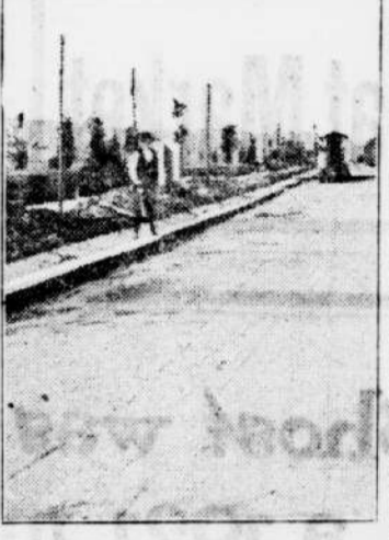
Construction of Concrete Road.
