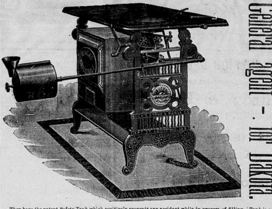
They have the patent Safety Tank which positively prevents any accident while in process of filling. Tank is convenient distance of the floor, being easily filled; this avoids the climbing on top of tables and chairs in order to fill the tank. It is impossible to fill tank while burners are lit.
